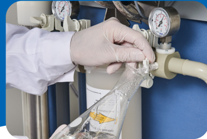
SDS 500 sanitary sampling port
